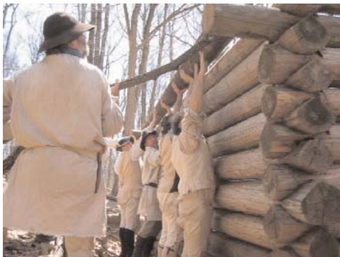
Volunteers repairing Pennsylvania Line Huts, NPS Photo
