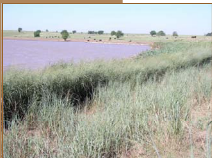
Vegetated berm of a flood control dam, Rice County, Kansas
