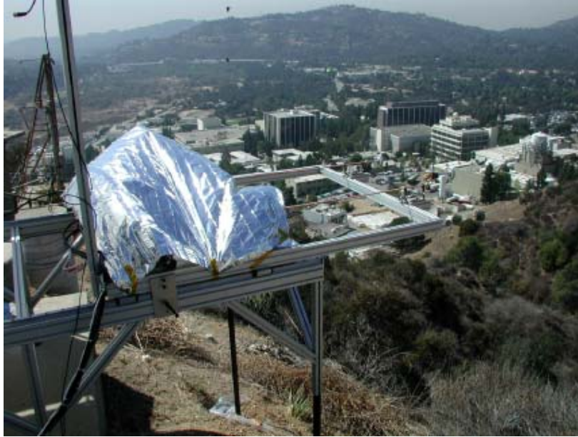
Fig. 8. The AFF sensor radiated test for end-to-end functional verification.
