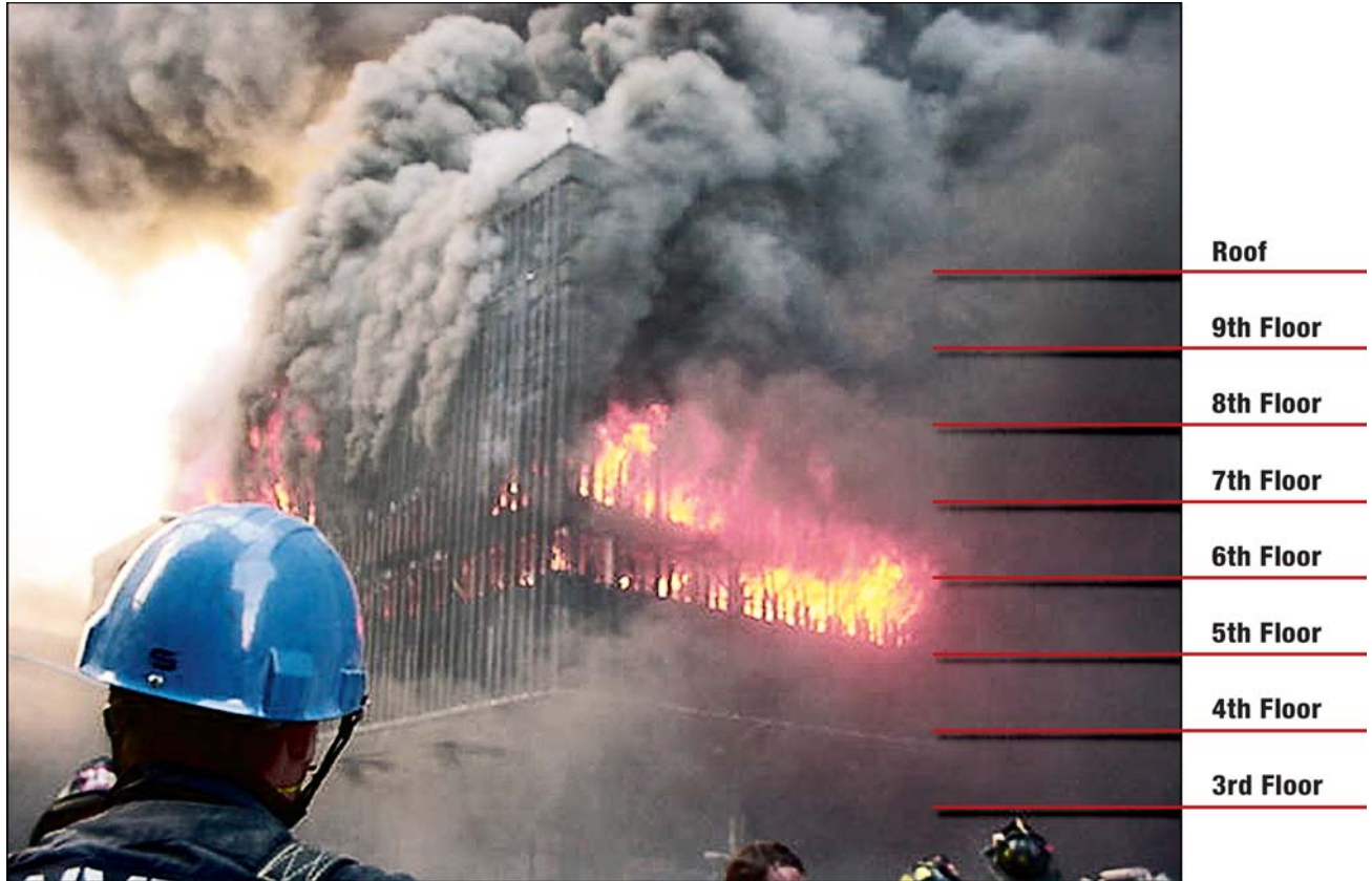
Figure 4-13 WTC 5 on fire.
