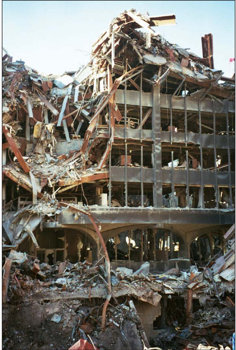
Figure 4-10 Impact damage to the exterior façade of WTC 6.
