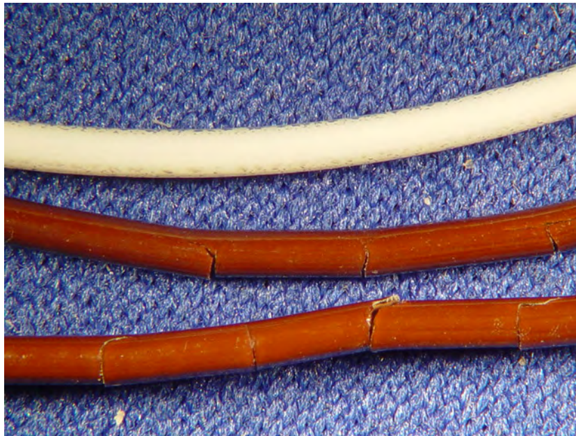
Figure 62. Unaged PV Wire (Top) and Aged Wires (Bottom) for 560 and 640 Hours
