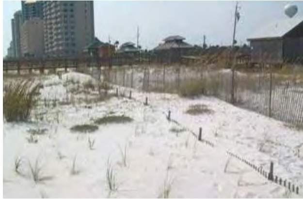
Primary and secondary sand fence.
