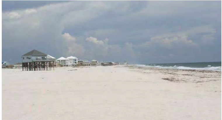
Loss of dunes leaves structures vulnerable to storm damage.
