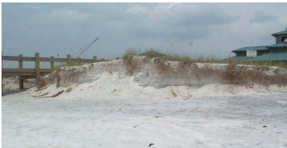
Dune front at Ft. Walton Beach, FL, lost during Hurricane Ivan in 2005. The buildings were not damaged.
