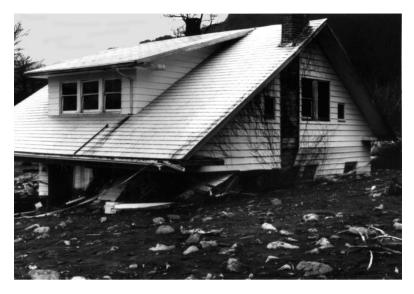
Figure 1 The west Dodson debris flows of February 8, 1996, entered this house situated on a fan at the mouth of a canyon about 60 km east of Portland, Oregon, and carried away owners' possessions without knocking the house from its foundation. This exemplifies the mobility of deforming debris-flow mixtures.
