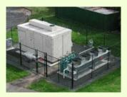
The fuel cell is interconnected to the school's electrical, heating boiler, make-up air, and potable water systems. Before the installation of the fuel cell, natural gas was not available on site. Consequently, natural gas service had to be added as part of the installation.
