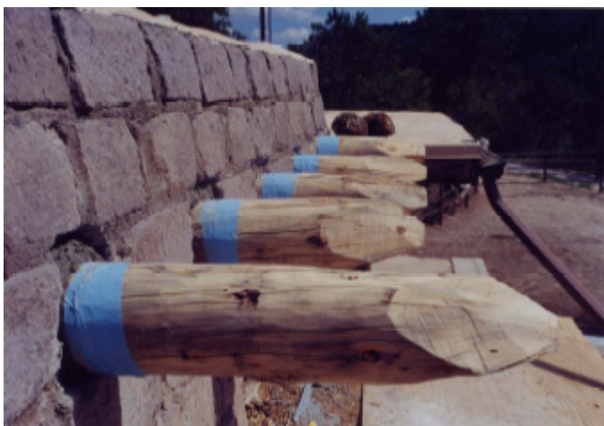
New viga ends threaded in place
