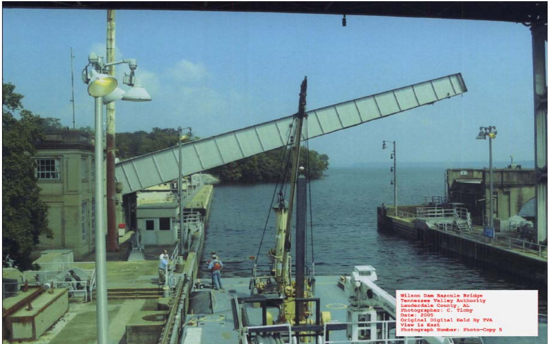
Figure 6. Bascule Bridge Opened Allowing for Barge Passage
