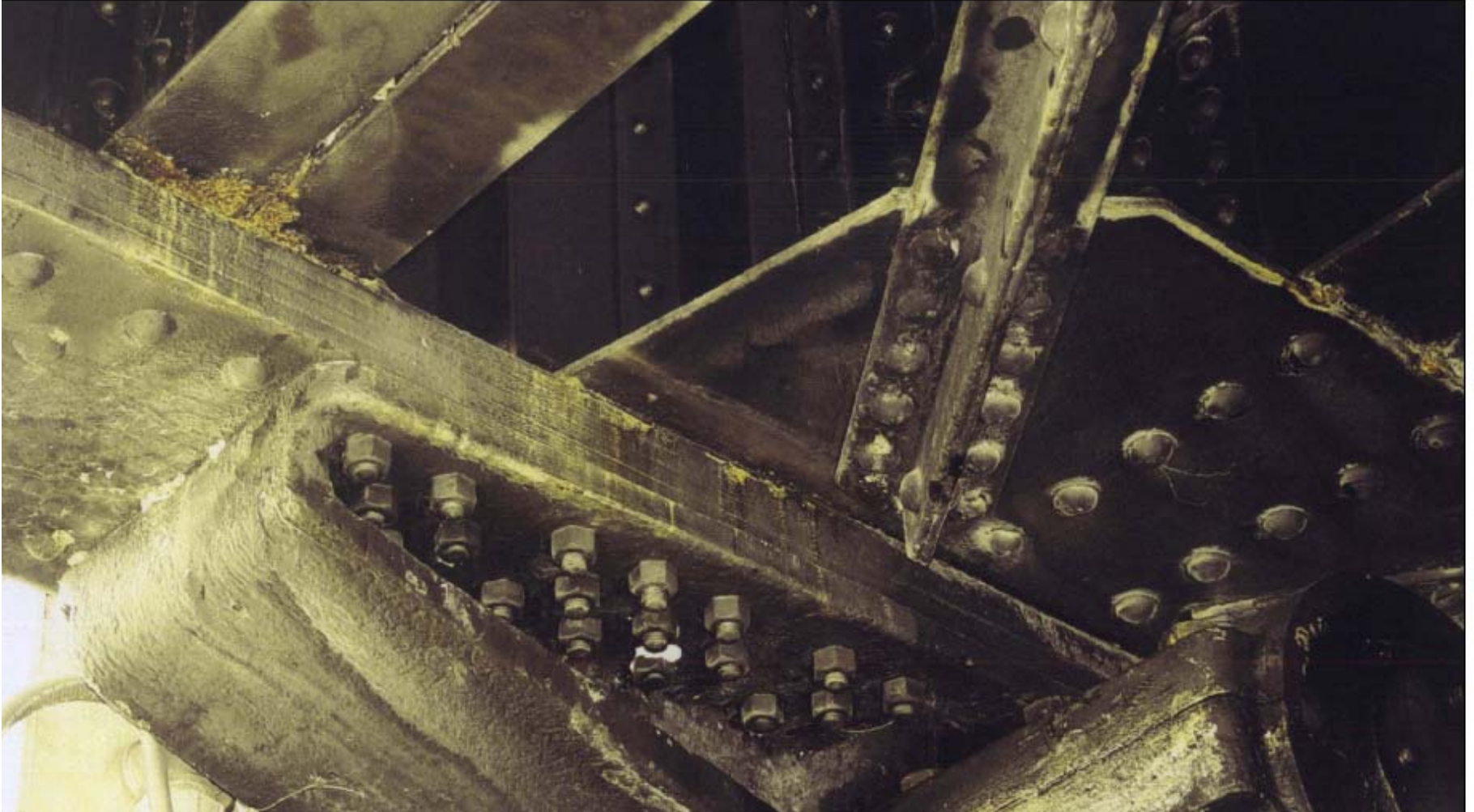
Figure 7. Photo of Current View Under Bascule Bridge
