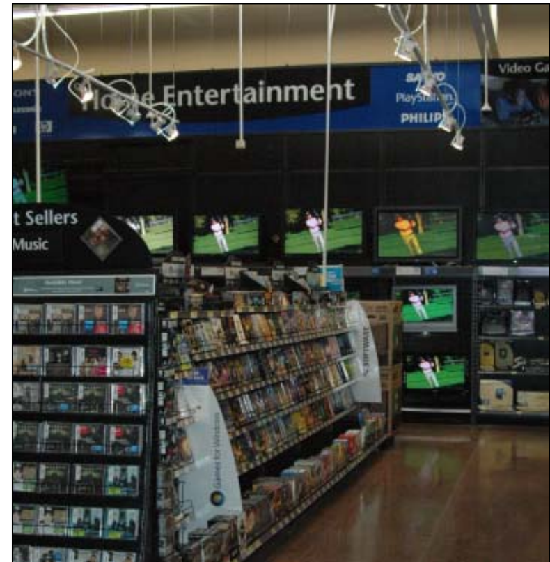
Installation at WalMart Store (TX) – Tracking sales under HSL every 15 minutes
