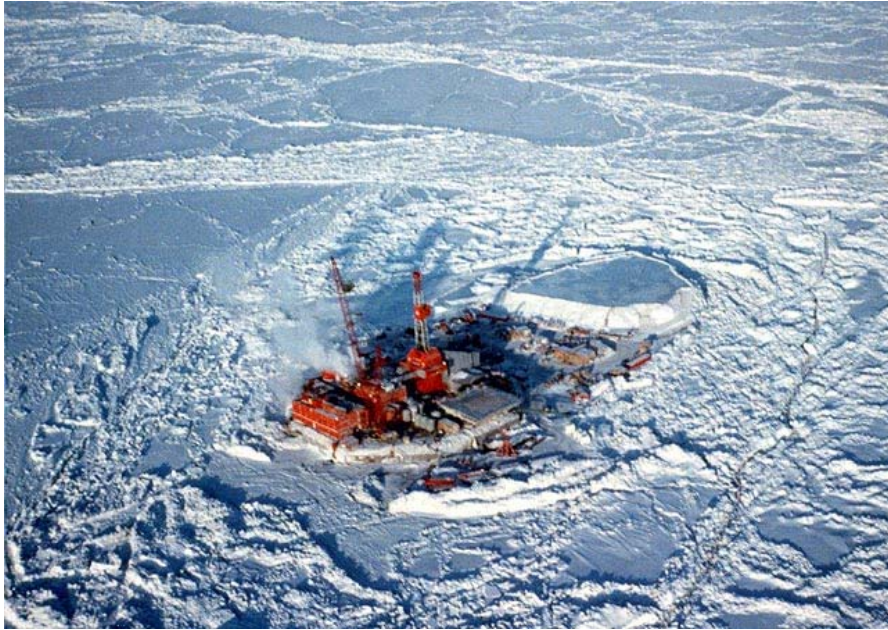
Figure 5.7: Tarsuit Relief Spray Ice Island (ICETECH, 2005)
