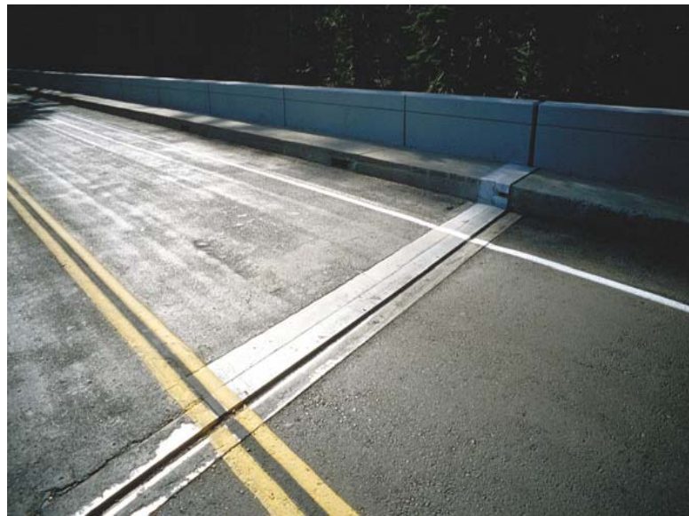
REMOVED AND REPLACED DAMAGED BRIDGE EXPANSION PLATE
