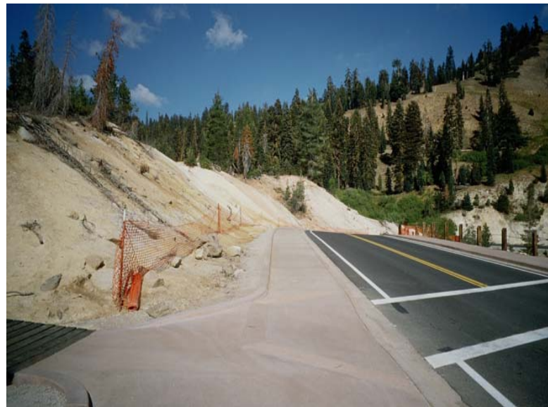
IMPROVED PEDESTRIAN ACCESS WITH NEW INTEGRAL COLORED SIDEWALK AND CURB/GUTTER
