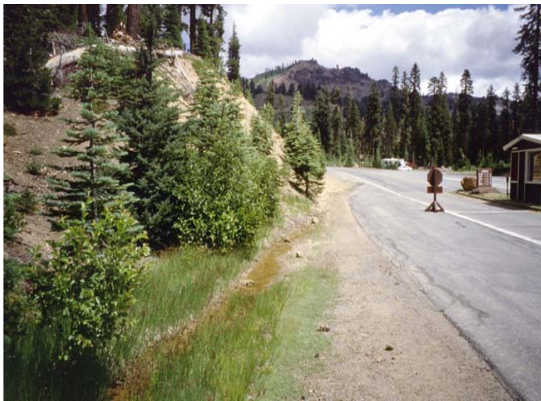
POOR DRAINAGE AND DETERIORATED ASPHALT
