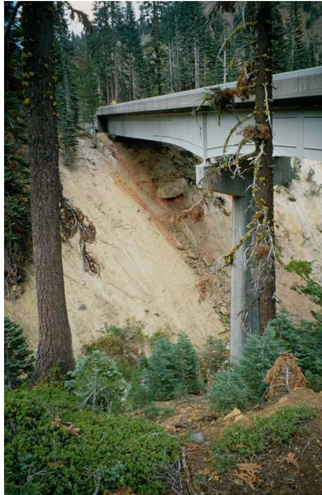
COMPLETED SLOPE DRAINAGE
