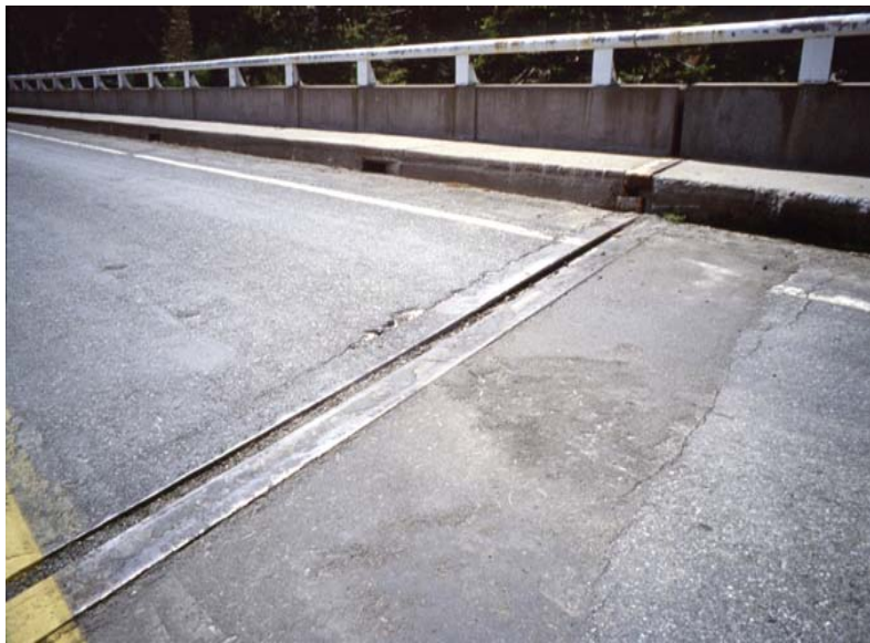
REMOVED AND REPLACED DAMAGED BRIDGE EXPANSION PLATE
