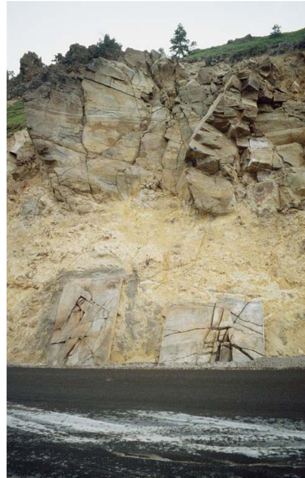
CARVED SHOTCRETE TEST PANELS AND PAINT APPLICATION
