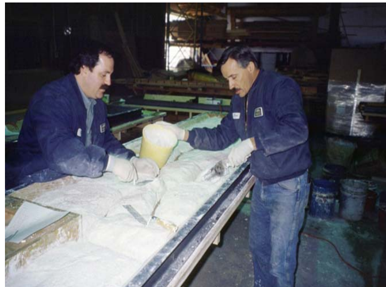
CONTINUING TO DEVELOP STONES WITH PLASTER
