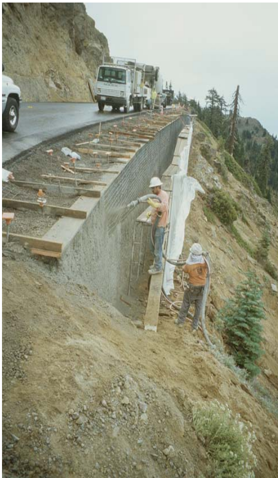
APPLYING SHOTCRETE TO MSE WALL
