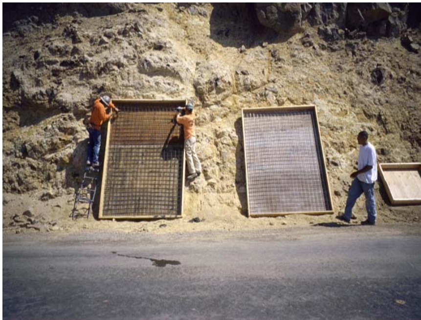
SHOTCRETE TEST PANELS
