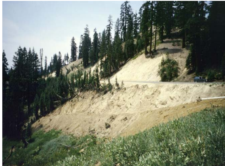
TOPSOIL PLACED
