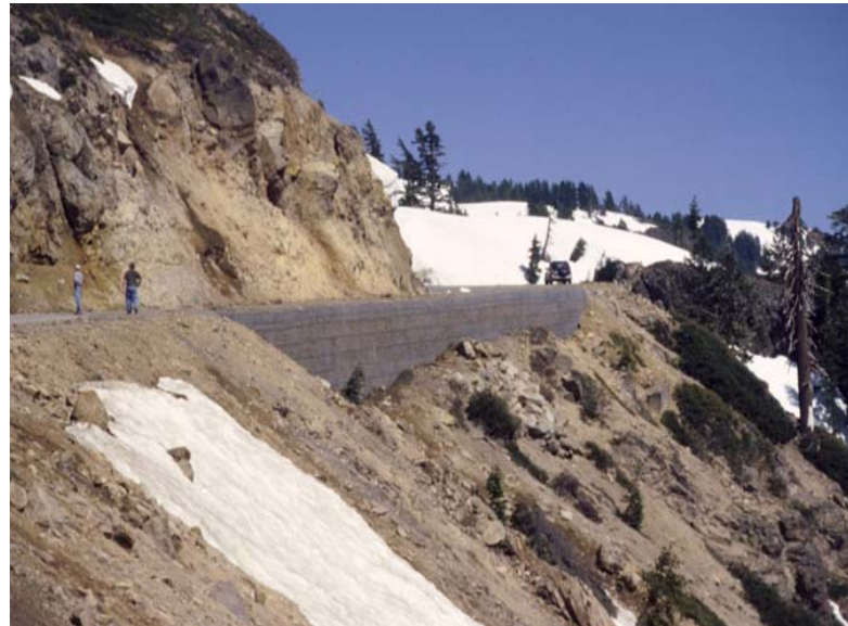
PRIOR TO CARVED SHOTCRETE APPLICATION
