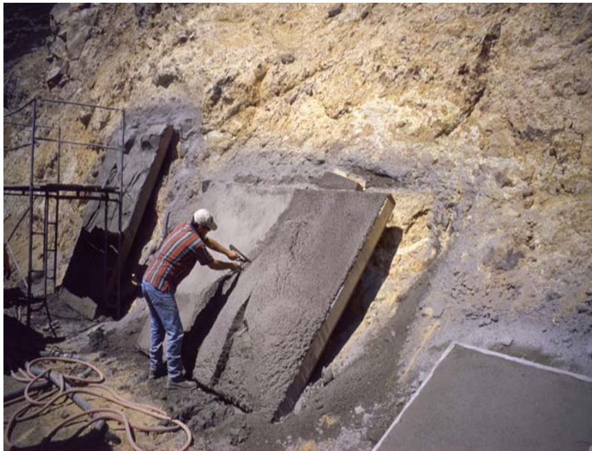
CARVING SHOTCRETE TEST PANELS
