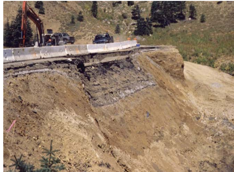
CLOSE UP OF SLIPOUT DURING CONSTRUCTION
