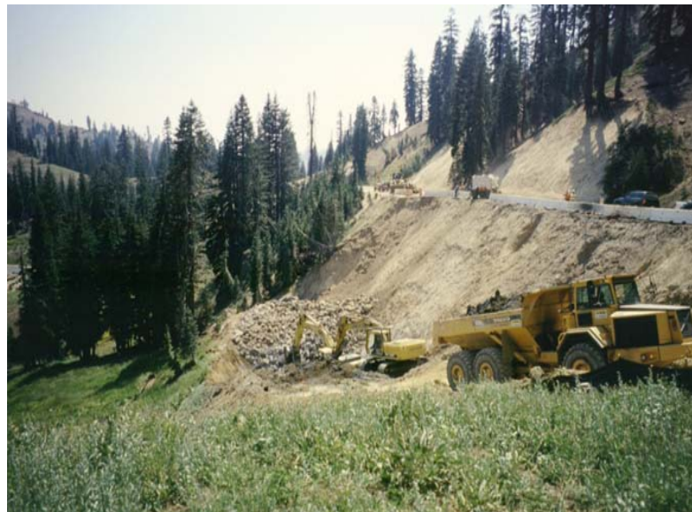
EXCAVATION AND PLACING ROCK
