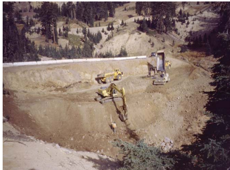
PLACING ROCK AND FILL MATERIAL
