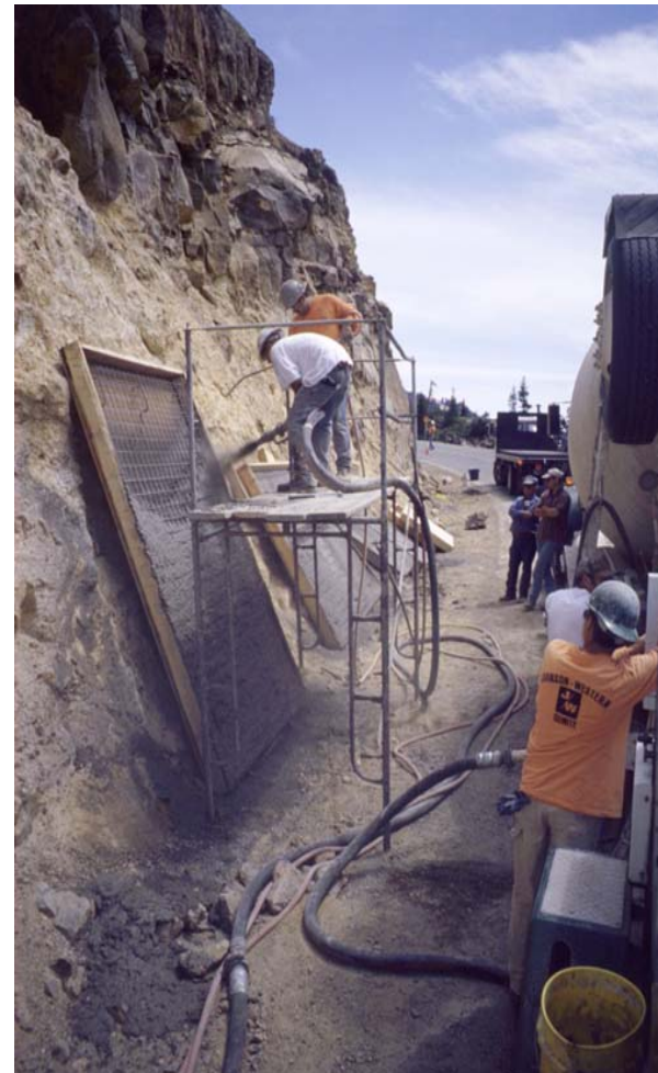
APPLYING SHOTCRETE TO TEST PANELS
