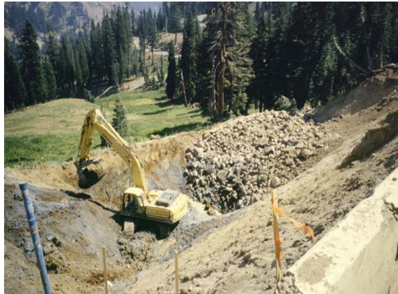
EXCAVATION AND PLACING ROCK
