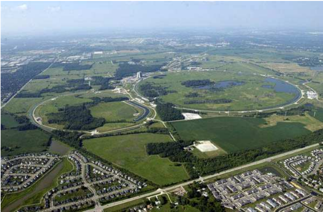
FIG. 2: An aerial view of Fermilab [31].
