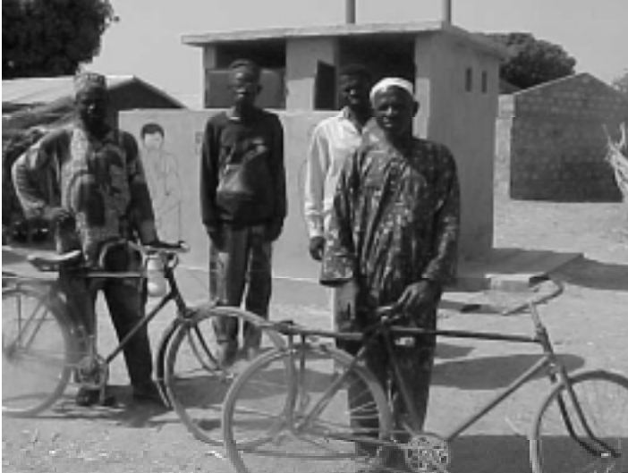
Figure 3. A GESCOME I CGMP in front of their GESCOME I latrine
