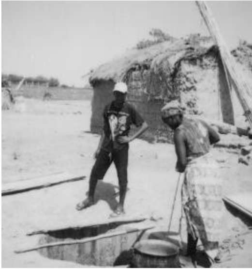
Figure 2. Unrenovated well, Banikoara
