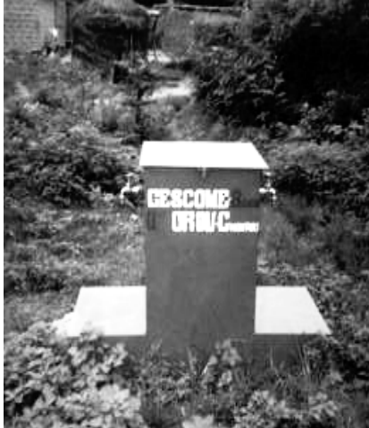
Figure 5. Latrine from an earlier development project that fell into disrepair and disuse, but was renovated by GESCOME.
