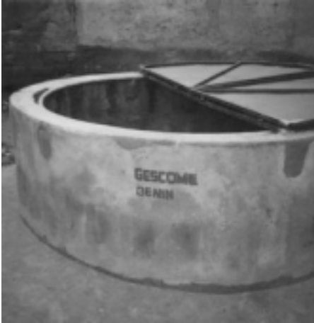
Figure 1. Gescome II well renovation, Demanou, Banikoara
