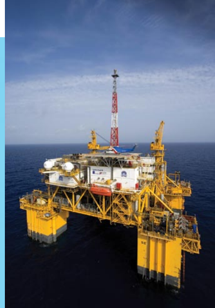
Figure 2. Anadarko's Independence Hub platform installed at the world-record water depth of 2,439 m. Photo Courtesy of Anadarko Petroleum Corporation
