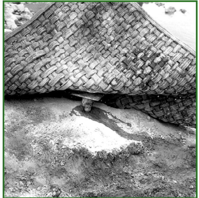
Figure 6—The blast mat is placed over the breech block.
