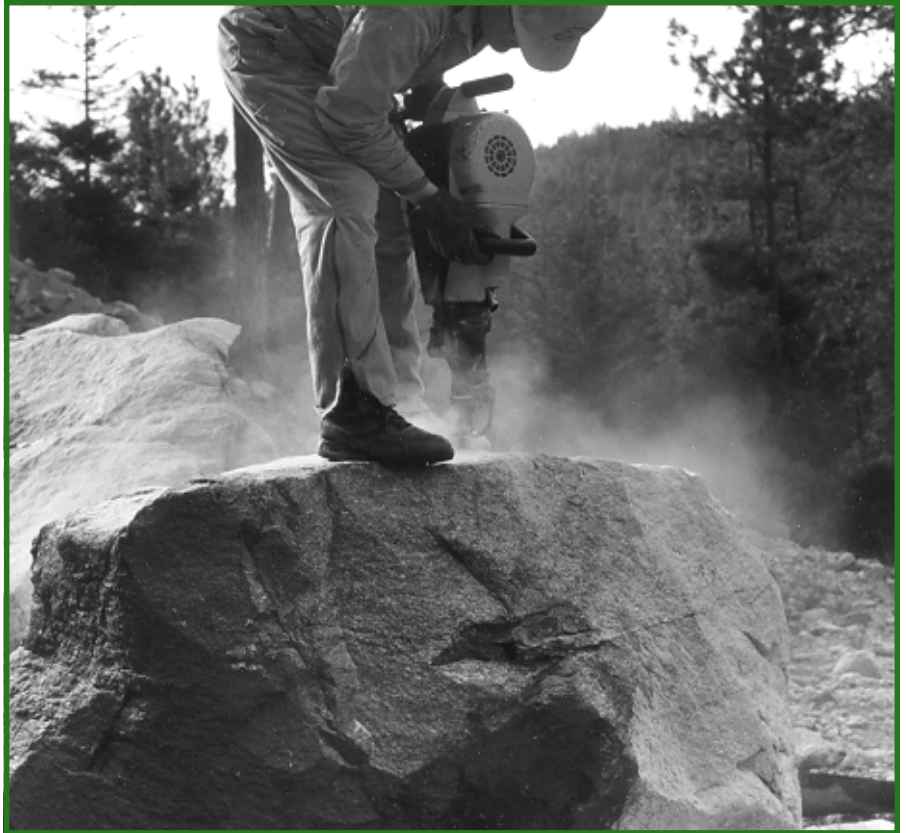
Figure 2—A hole is drilled in the boulder using a portable drill.
