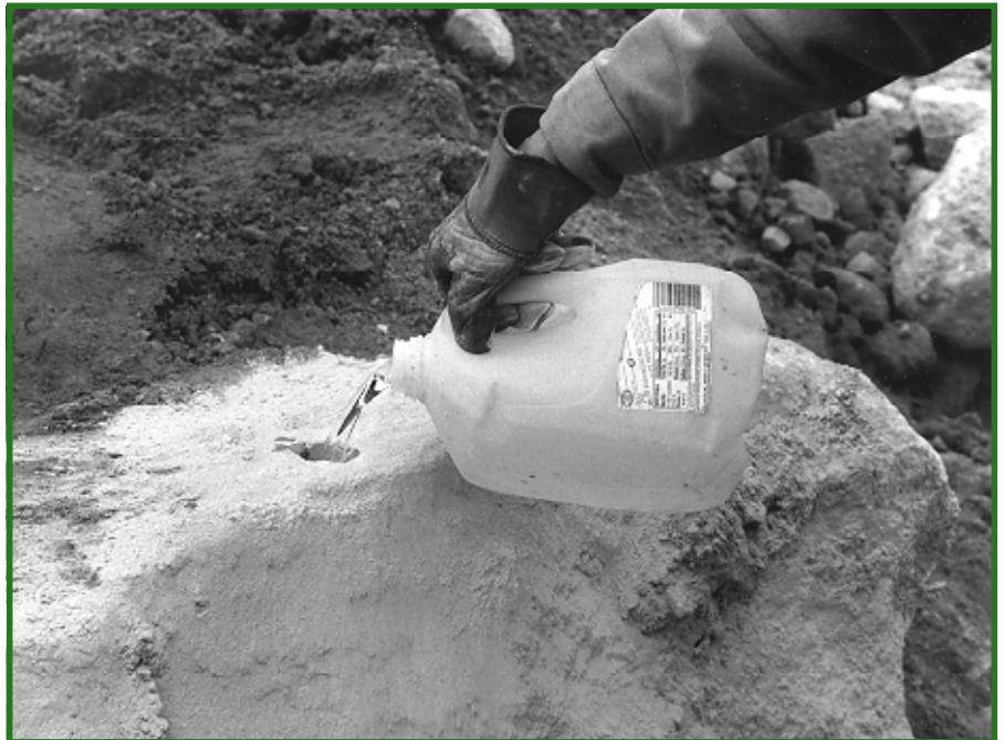
Figure 3—Water is poured into the hole.
