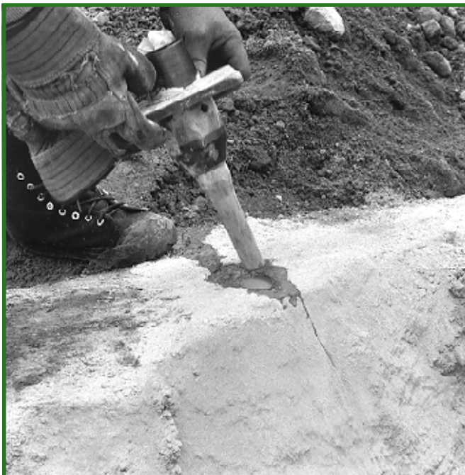
Figure 5—The impulse barrel and breech block assembly is placed in the hole.
