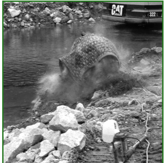
Figure 11—The lanyard is pulled to fire the primer cartridge.
