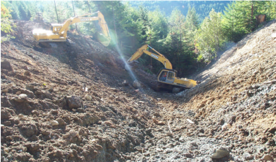
Pair of excavators
