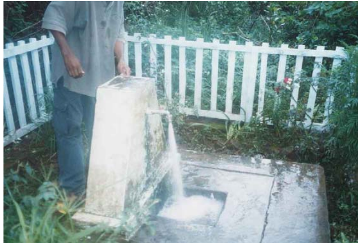
The street fountain #15 located at the tail of the water supply system
