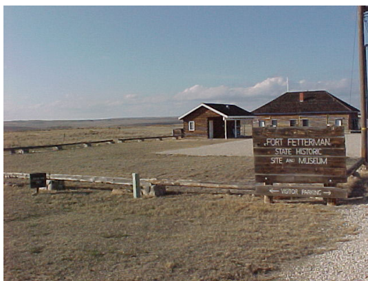
Top to bottom: Fort Laramie Cavalry Barracks, Fort Laramie National Historic Site, vicinity of Torrington, Wyoming; Wyoming Pioneer Museum in Douglas, Wyoming; Townsend Wagon Train Fight Site, Johnson County, Wyoming; Fort Fetterman, vicinity of Douglas, Wyoming. Photos by Christine Whitacre.
