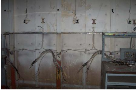
Figure 2 Typical space with peeling paint and bulkhead insulation.
