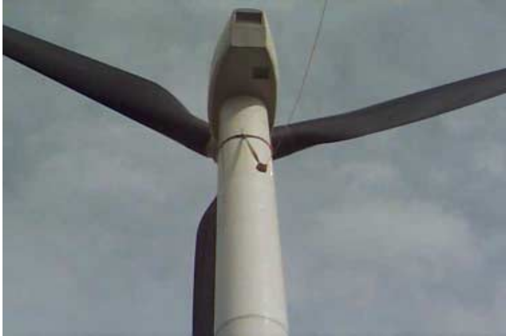
Figure 5. Step-relaxation load method applied to tower
