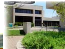
National Combustion Research Facility
