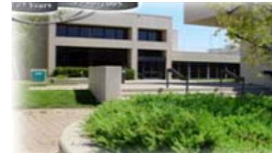
National Combustion Research Facility
