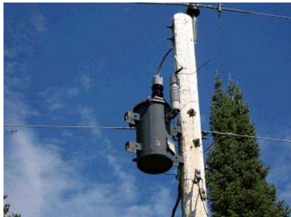
Removing PCB-containing transformers helps safeguard the environment from leaks or spills
