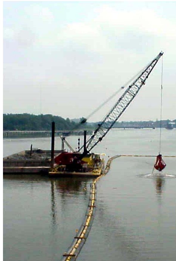
A sediment remediation project underway
