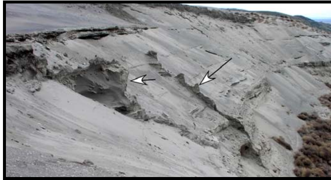
Figure 2.6. A Pair of Vertical Clastic Dikes (arrows). These dikes crosscut SD flood deposits exposed along the White Bluffs just east of the Hanford Site. The dikes stand out here because they contain more cohesive silt and are better able to withstand attack by strong winds, which are actively eroding these bluffs.
