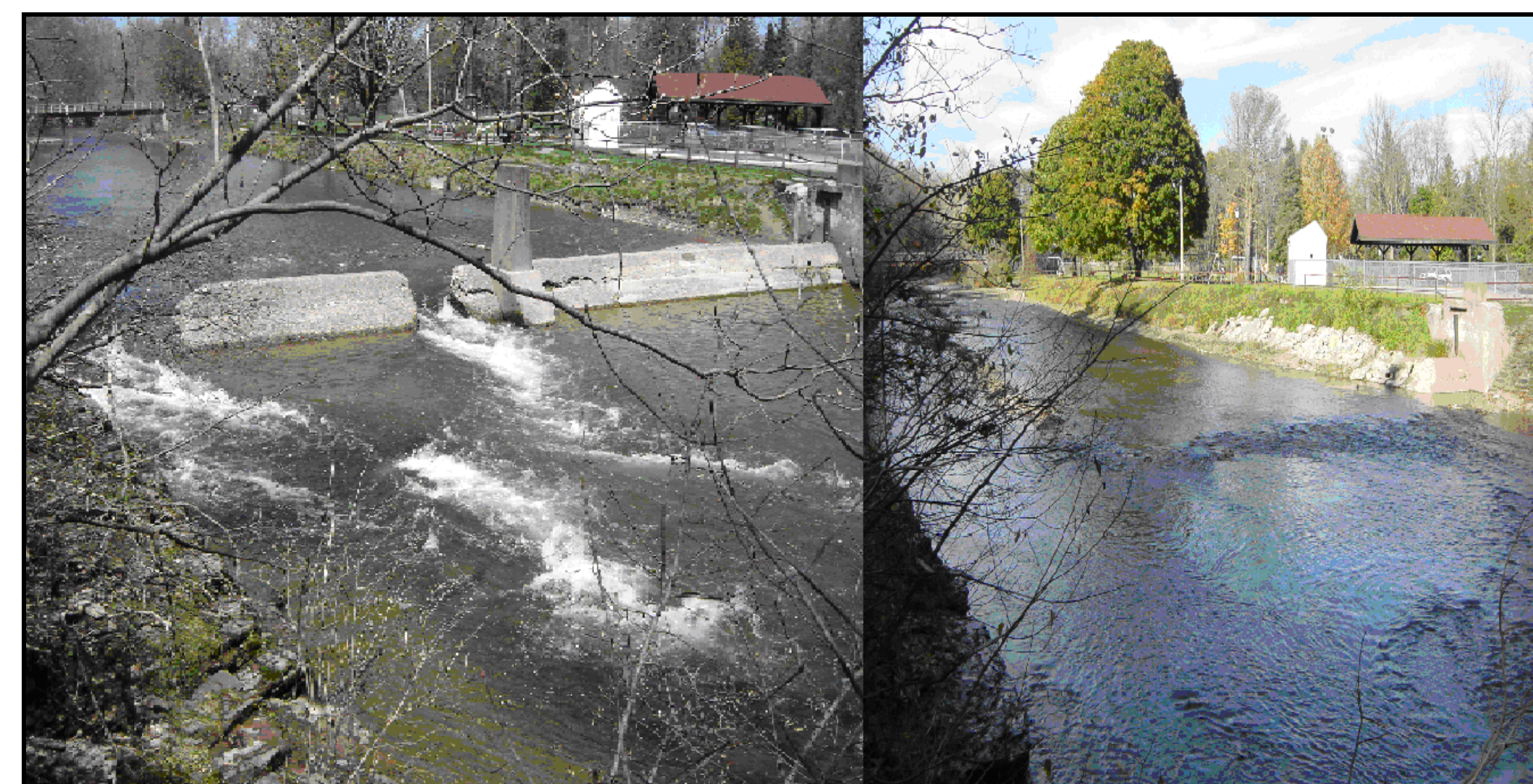
Before and after photos of the dam removal project in Canasawacta Creek. Credit: Raymond Li (USFWS)
