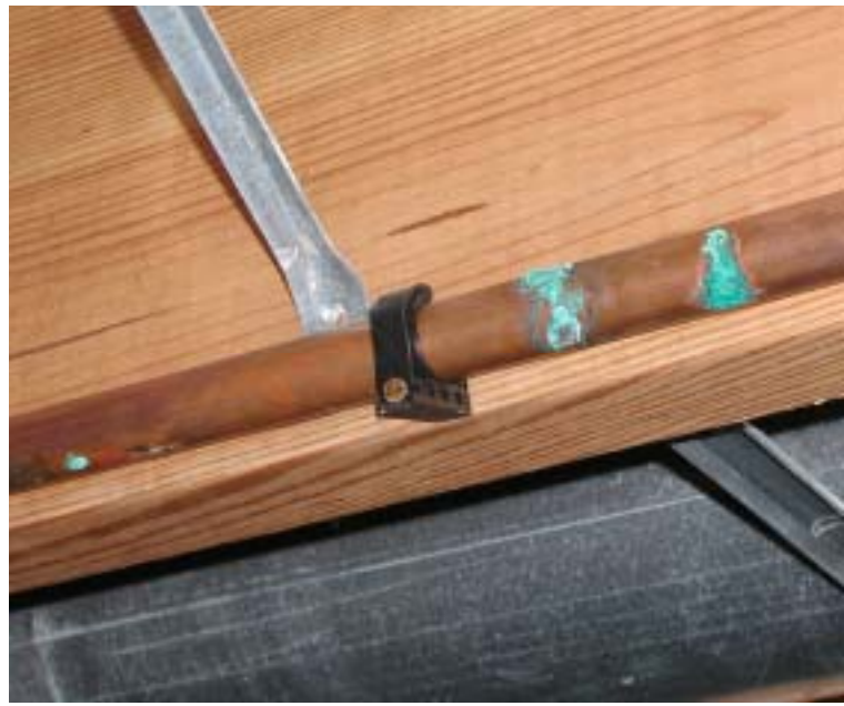
Pinhole leaks resulting from copper pitting
