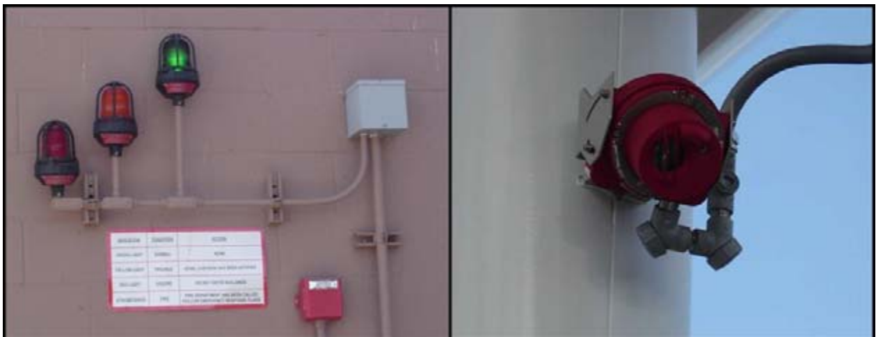
Figure C-5. Condition indicator lights (left) and hydrogen flame sensor (right) at the Chevron – AC Transit Hydrogen Energy Station
