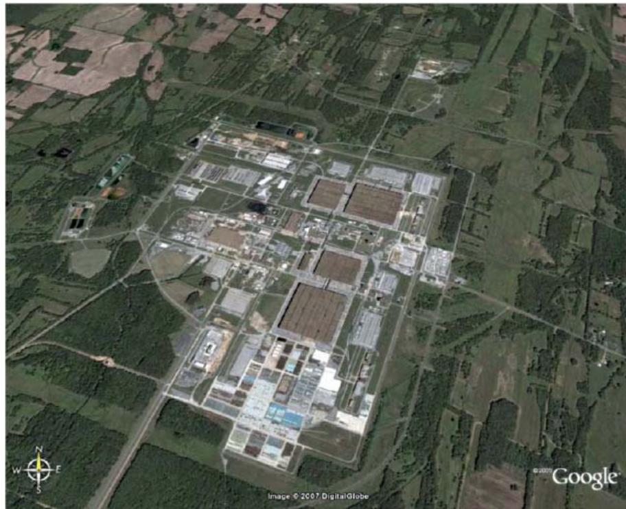
Paducah Gaseous Diffusion Plant (PGDP) Paducah KY
