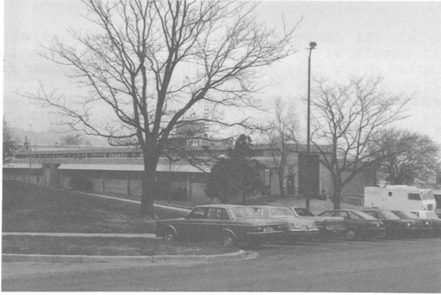
Figure 3. Wing 4 of the Radio Building with ITS millimeter-wave measurement van.
