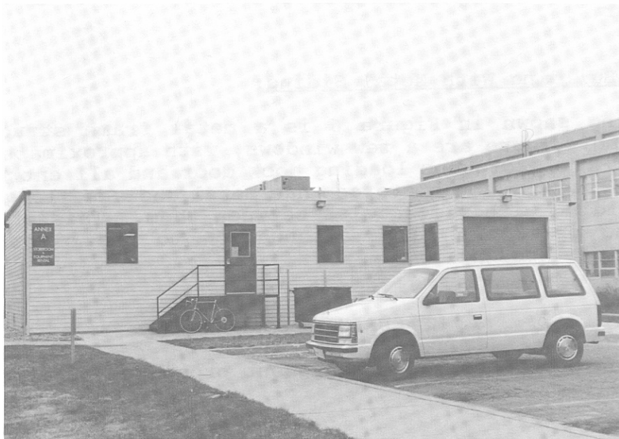
Figure 6. Storeroom with metal siding.
