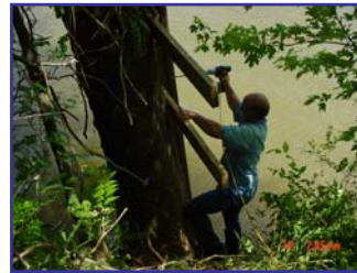
Data Acquisition Program Manager Larry Dattilo installing a new river gauge.
