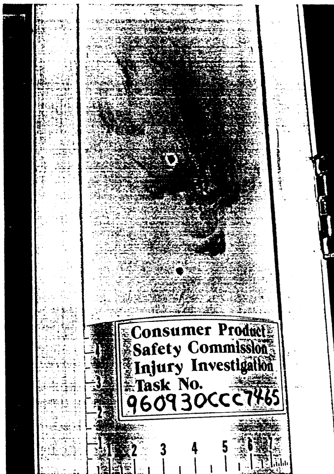
PHOTO #1: Close-up photograph of the area on the wall in the hall, where the smoke detector had been mounted. The consumer reports that this area on the wall was washed, after this fire.
