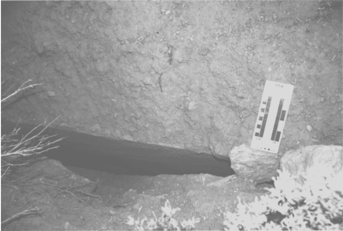
Figure 12. U-19ab (Towanda). Newly opened crack in bedrock covered by a veneer of soil. Such cracks may follow preexisting joint patterns in the bedrock, but to show this much fresh opening, require recent ground motion of large amplitude.
