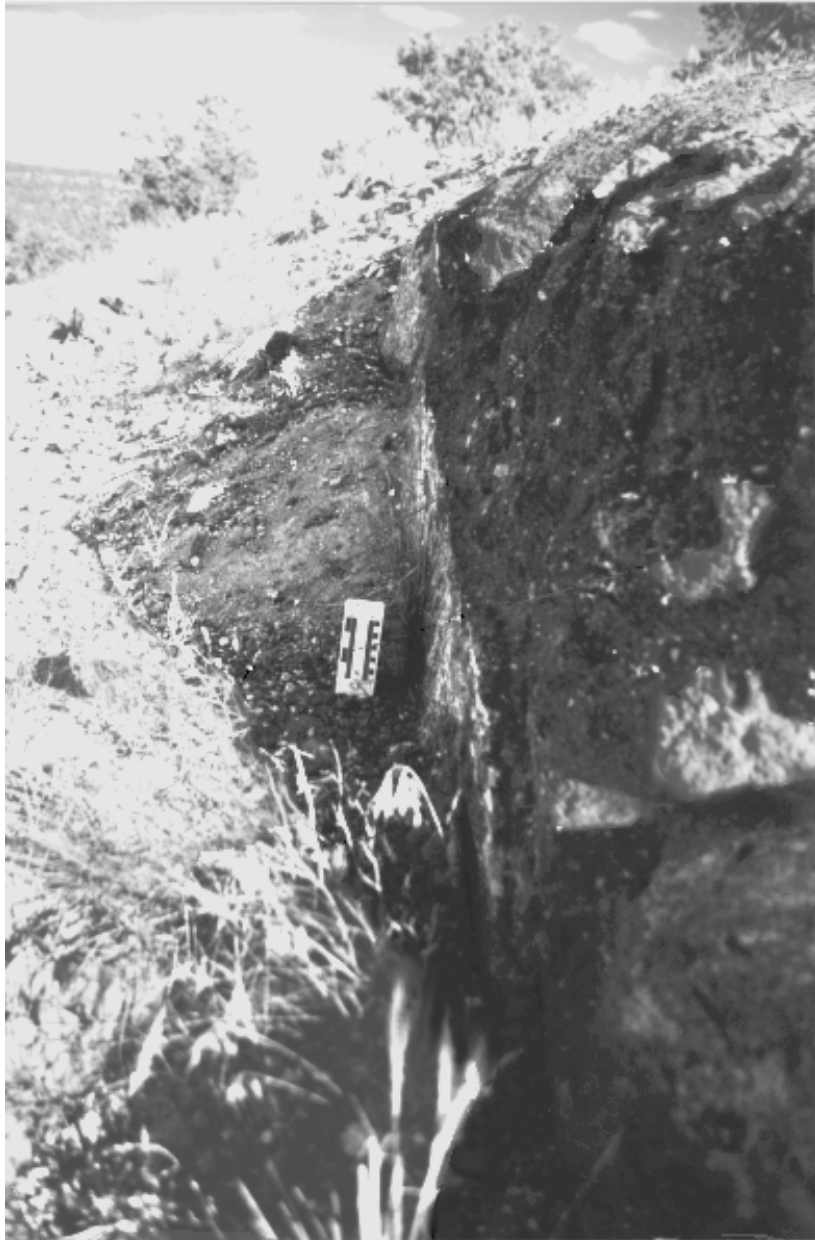
Figure 9. Crack in bedrock showing offset downward toward the area of prepared ground and presumably SGZ. Note the 10-cm ruler for scale.
