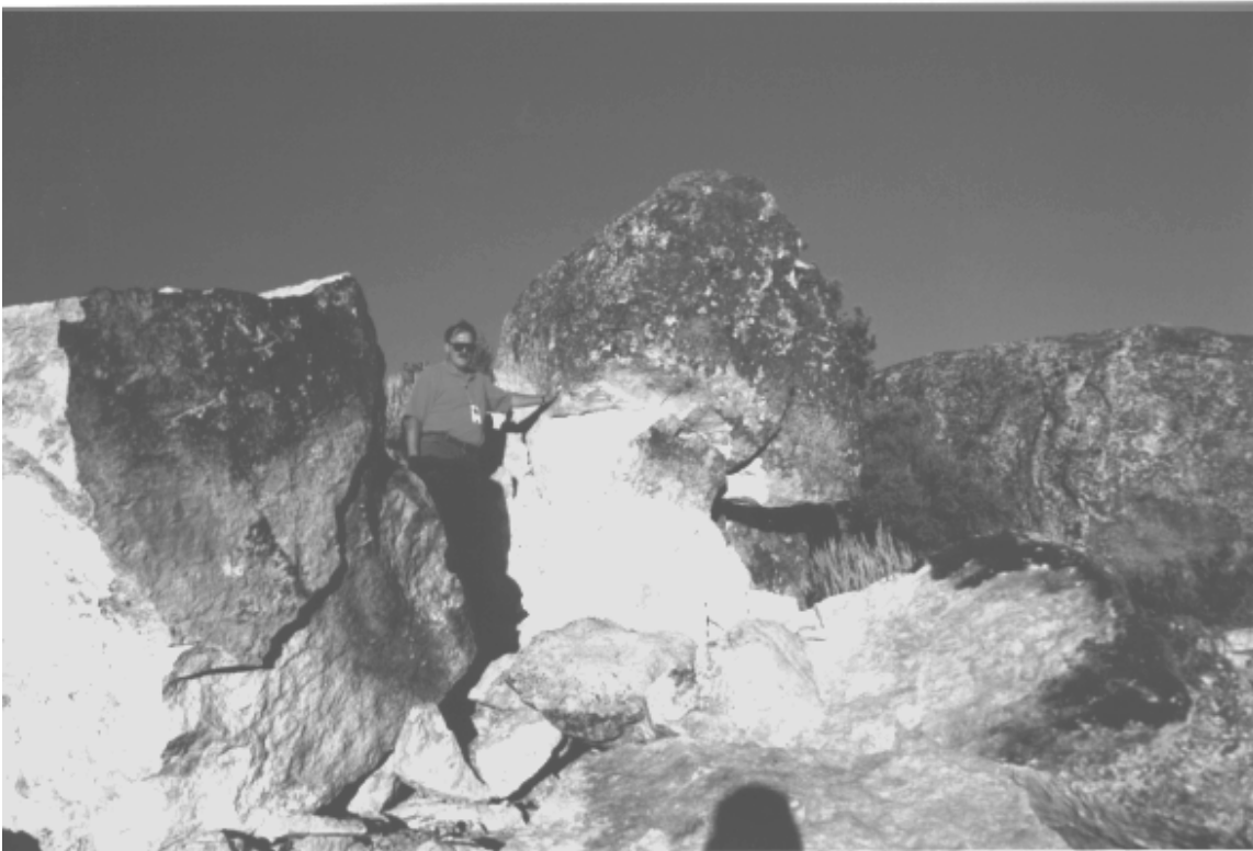
Figure 11. Block spall along low cliff near perimeter fence of Towanda. Note the light-colored fracture surfaces (fresh) in contrast to the darker (old) surfaces.
