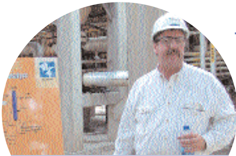
A Silver Eagle Facility Manager introduces a new energy-saving catalyst technology at the 2001 Utah Showcase
