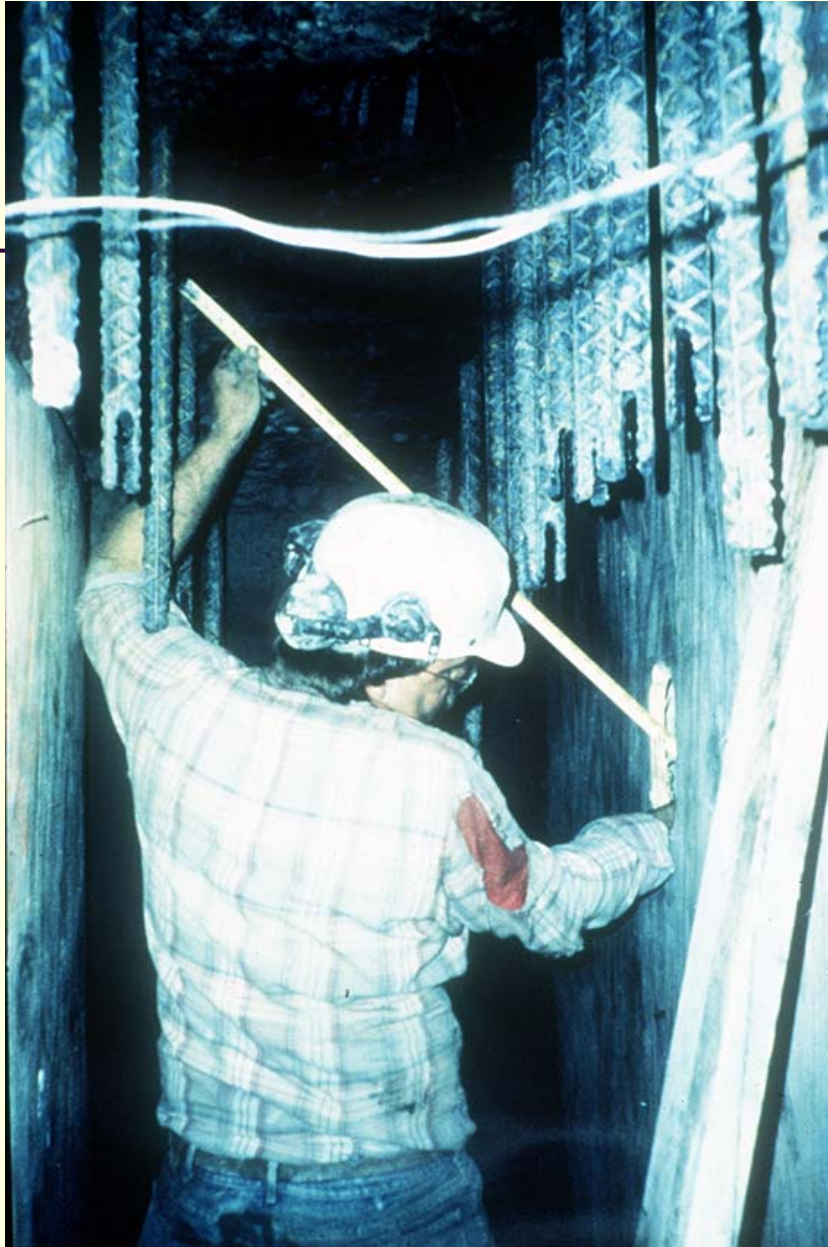
Roof Dowels for Anchorage
