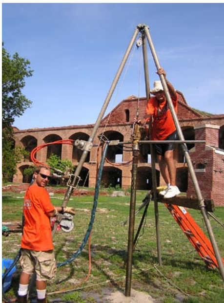
Drilling a well at Fort Jefferson. Gene (right) operates the drill. Don is on the winch.
