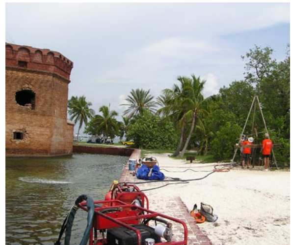
Installation of another well in the transect.
