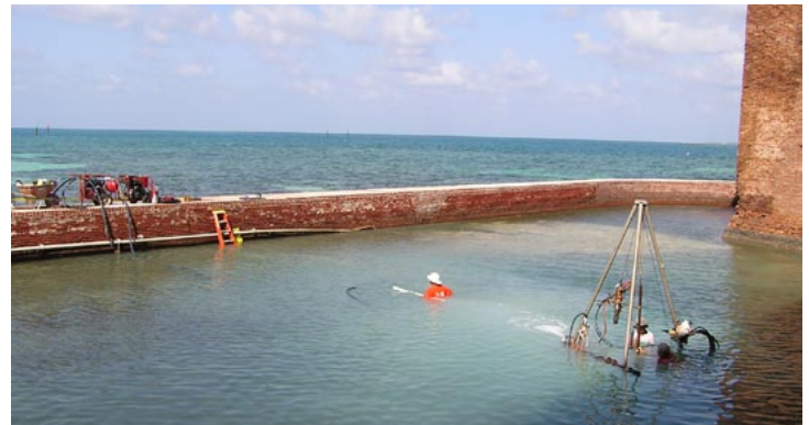
Carrying core inside a core barrel to the moat wall.
