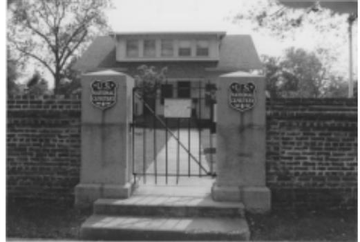
The lodge, constructed in June 1916 of wood frame and stone, is two stories and contains six rooms. The roof is asphalt shingles. Aluminum siding was installed on September 3, 1960. There is a partial basement, and an office is maintained on the first floor. The entire second story was remodeled in 1932 to add a bedroom, alcove, and bath. There is a roof over the entry on the northeast side of the lodge. The dormer has a sheet copper roof. The windows are double-hung.
