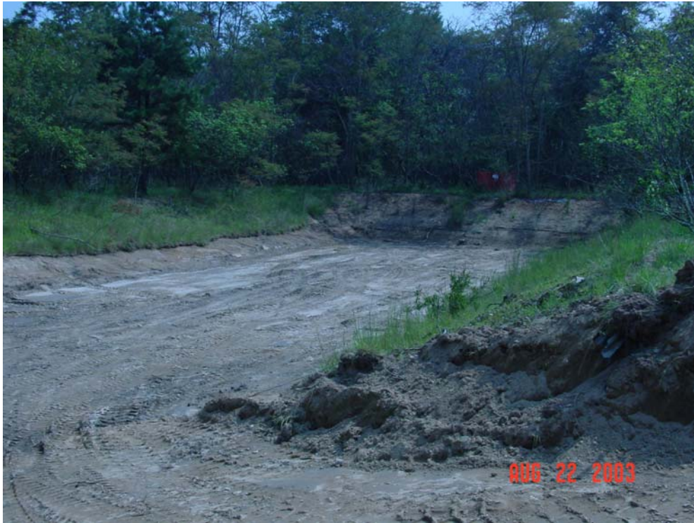
Figure 5: East Pond Following Sediment and Liner Removal
