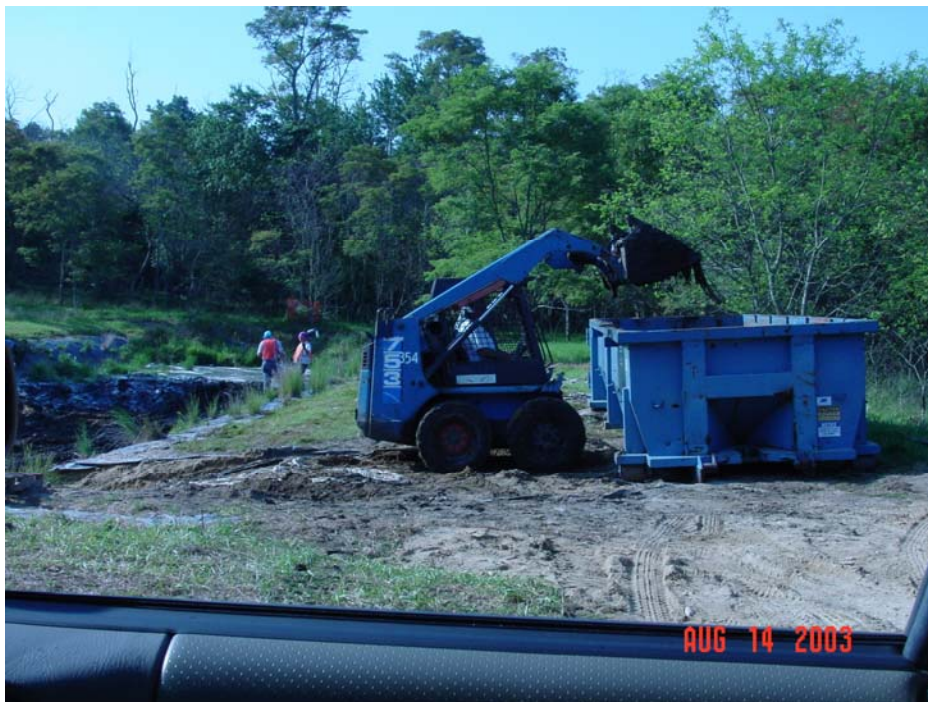
Figure 4: Bobcat Placing Sediment in Roll-off Container
