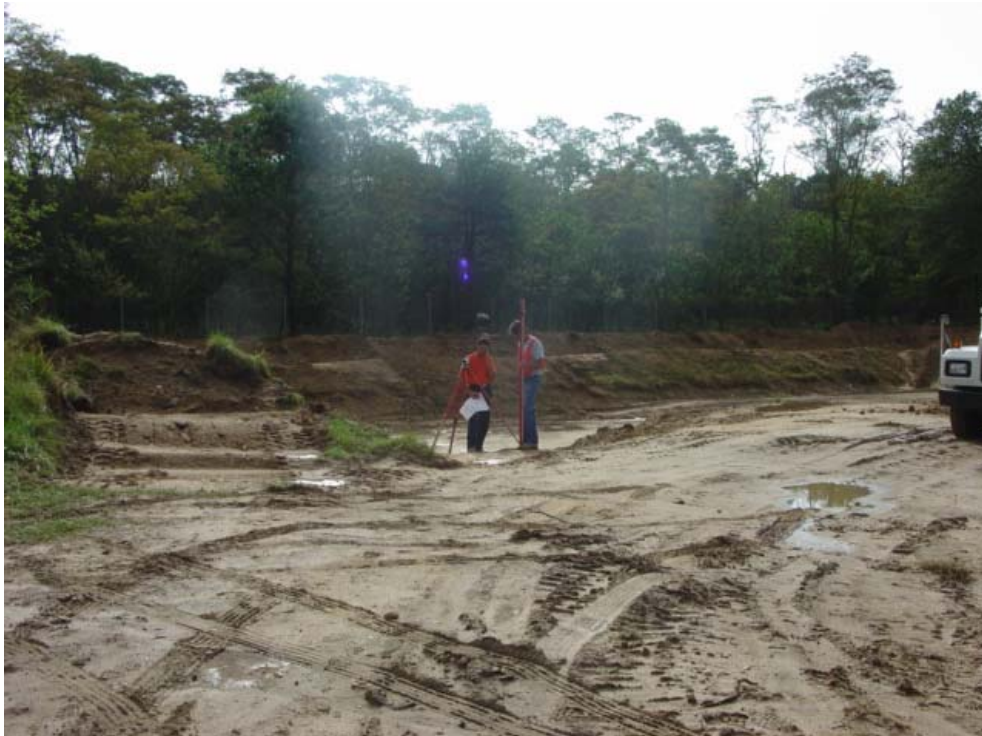
Figure 8: Land Surveying for Proposed Pond
