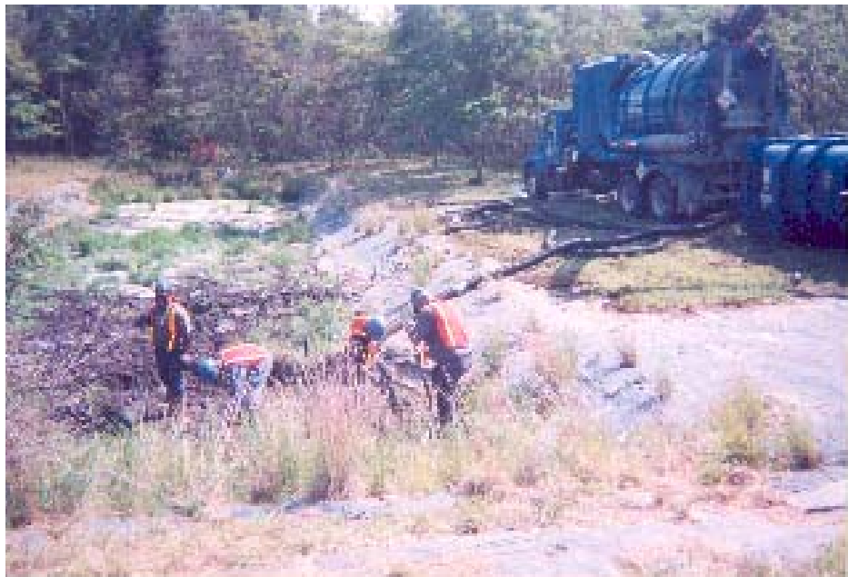
Figure 2: Removal of Sediment with Vacuum Truck
