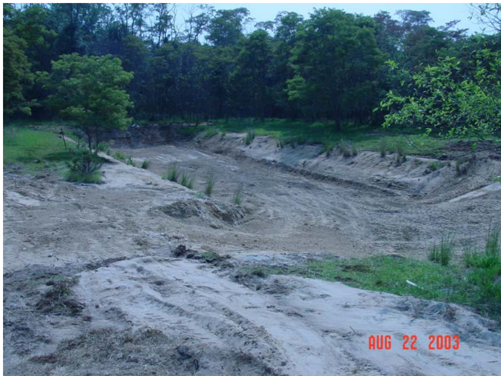
Figure 6: West Pond Following Sediment and Liner Removal
