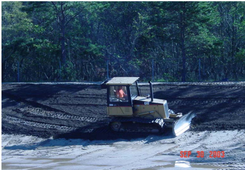
Figure 10 Placement of Top Soil in Pond
