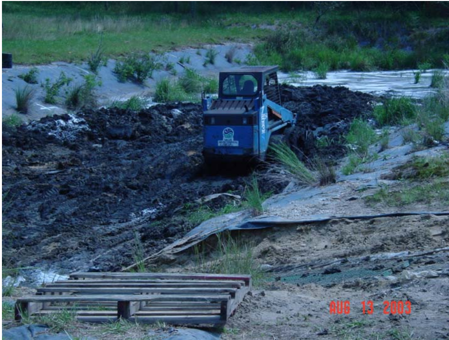
Figure 3: Removal of Sediment with Bobcat
