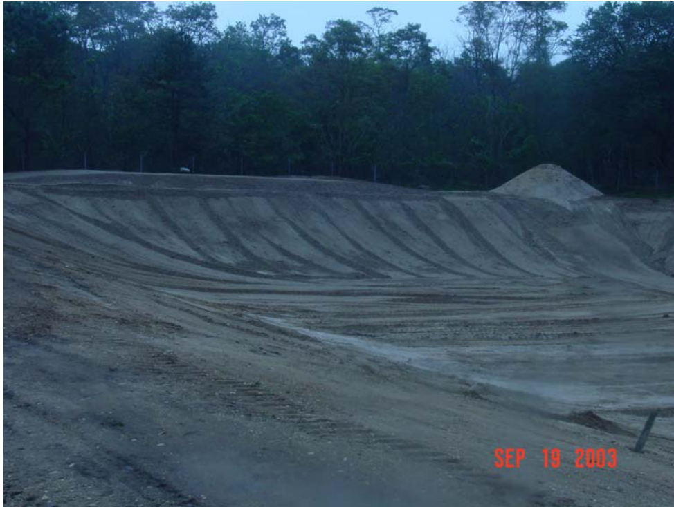
Figure 9: Graded Pond Prior to Liner Installation
