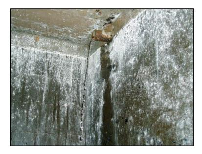
Figure 14. Inflow to the cistern at Split Rock Spring through 2-inch diameter steel pipe near the cistern ceiling.
