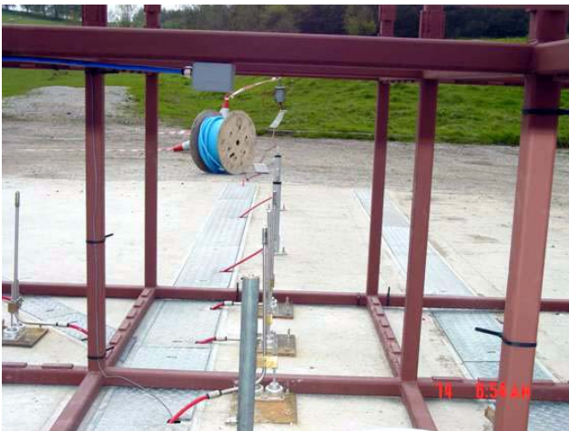
Figure 3. Testing Sensors with Igniter
