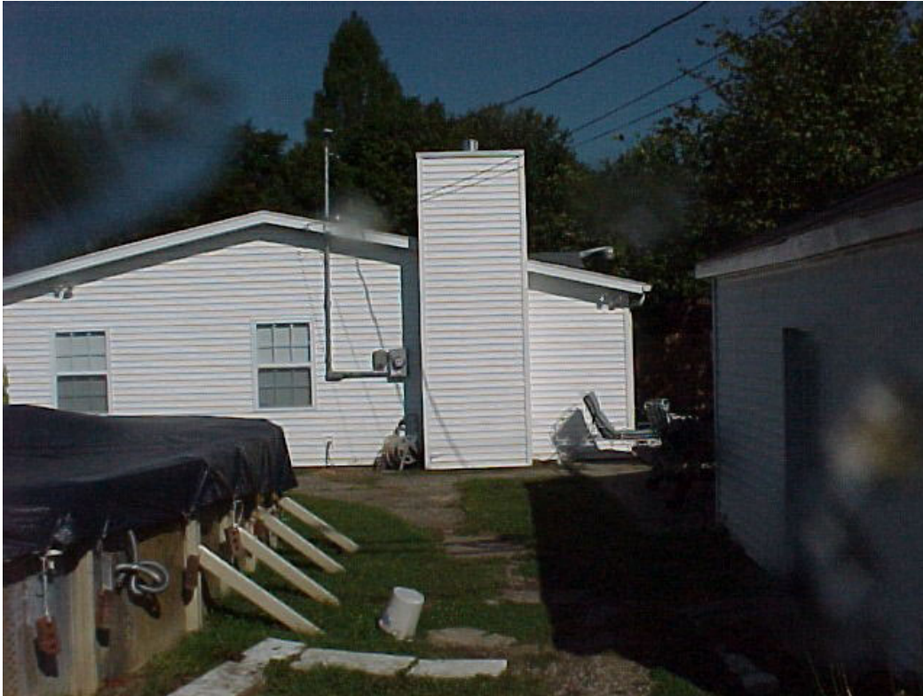
Photograph. Residential structure involved in the incident
