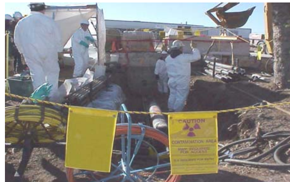
Preparing to begin drilling and sampling operations
