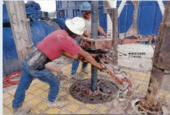
Fig. 9. Breaking out drill pipe
