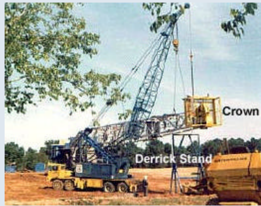
Fig. 5. Setting crown on derrick stand
