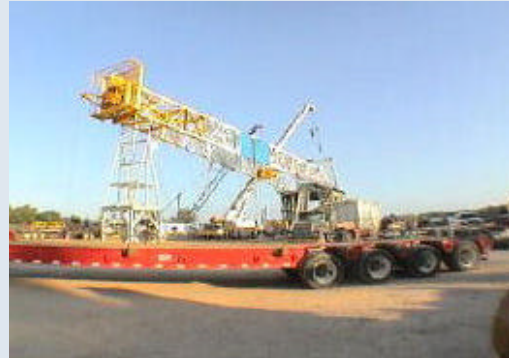
Fig. 6. Rigging up the mast
