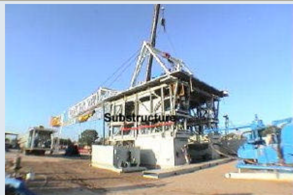
Fig. 2. Setting up the substructure
