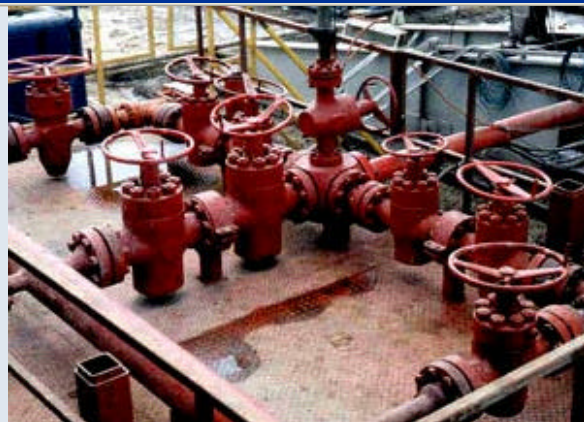
Fig. 5. Choke manifold
