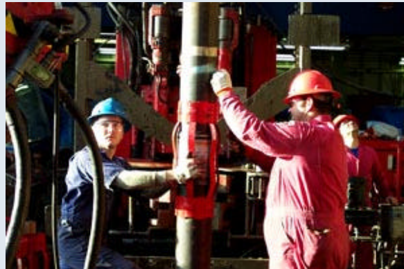
Fig. 7. Installing casing centralizer
