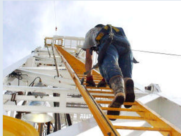
Fig. 6. Climbing Assist Device and PPE
