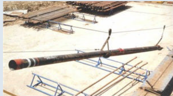
Fig. 4. Lifting casing onto rig floor
