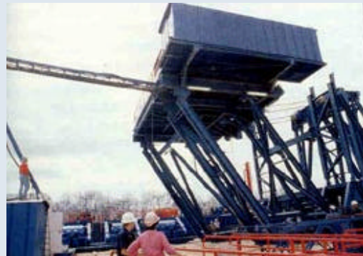
Fig. 3. Raising the doghouse and rig floor
