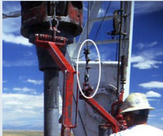
Fig. 4. Improper wire rope clamp placement "Never saddle a dead horse"
