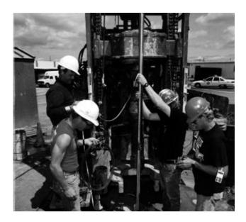
Dynamic underground stripping combines steam and electrical heating of underground soils with vacuum extraction of vapors and fluids, guiding these processes by real-time monitoring methods.
