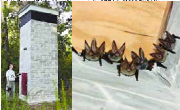
"Concrete trees" like this one in Texas were designed by Bat Conservation International to simulate the large tree hollows that some forest bats require for roosts. This one was occupied within months by Rafinesque's big-eared bats.
