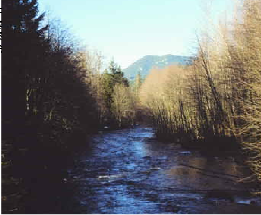
Large streams provide foraging and drinking habitat for bats. I-beam style concrete bridges and bridges with vertical crevices (expansion joints) can provide ideal roosting sites when they span such streams.
