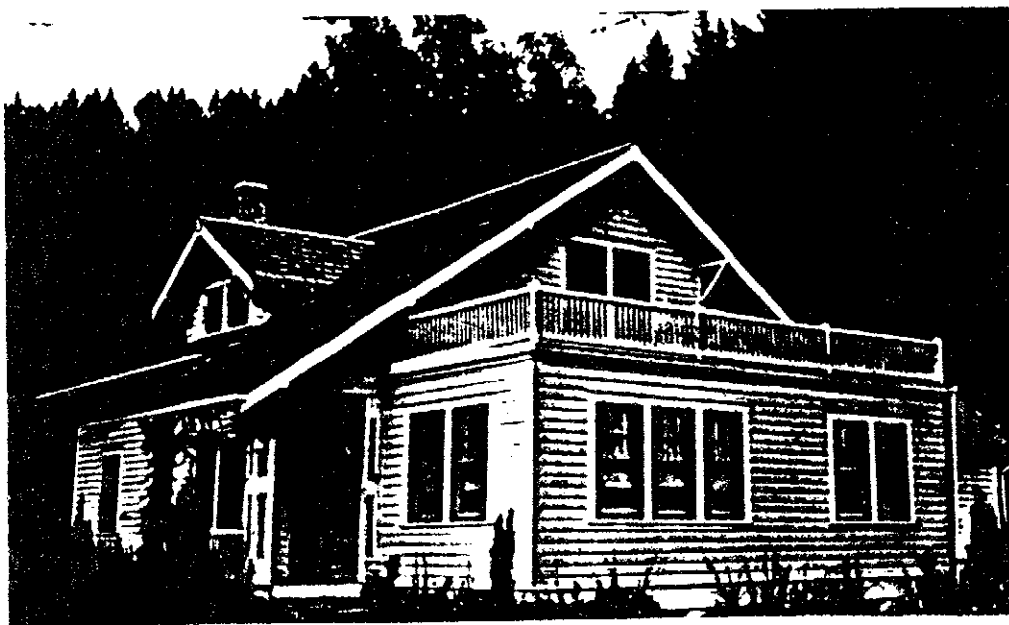
1937 photograph showing the 1936 addition to east side of Randle Ranger Residence. View is to NW.
