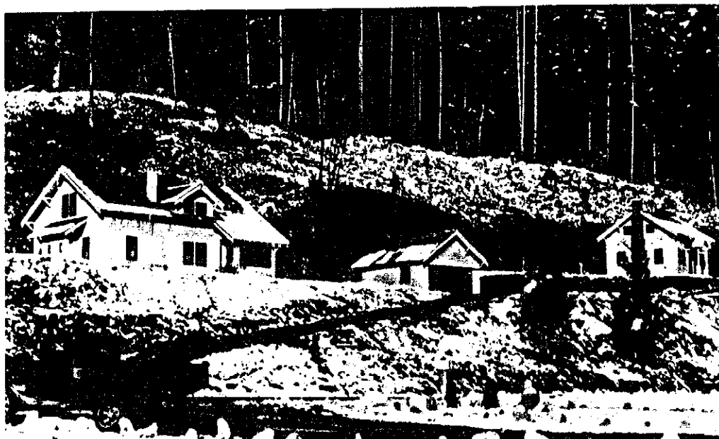
1935 photograph of Randle Ranger Residence (left), associated garage and Protection Assistant Residence (right). View is to NNE from junction of Silverbrook and Slagle Roads.
