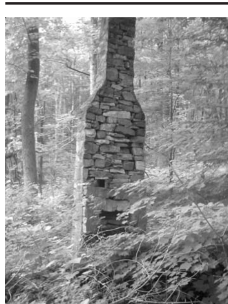
Intact chimney at 2EX441.
