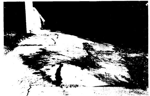
SHIFTING EARTH-Surface faults in the Houston area sometimes cause extensive damage to houses and commercial buildings such as this cracked driveway and distorted house on Billings Street. A homeowner with damage from surface faulting is usually stuck with an unsaleable or greatly devalued house.
