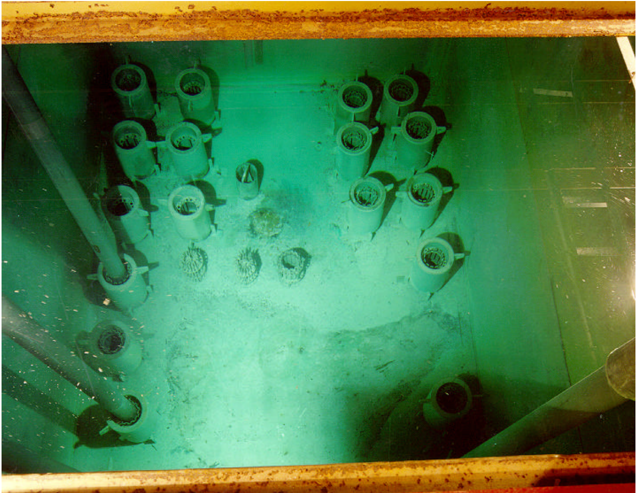
Figure 6 View of sources with tubes removed.
